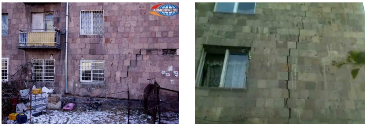
Fig 2. 4th class emergency buildings to be demolished in Yerevan
