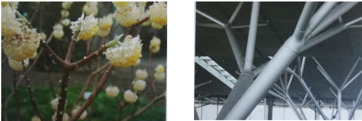
Fig. 1. Detail of the ramification of the Oriental paperbush ( Edgeworthia chrysantha ), with three branches of almost identical diameter (left), and branched columns at Stuttgart Airport each with three or four equivalent struts (right)
