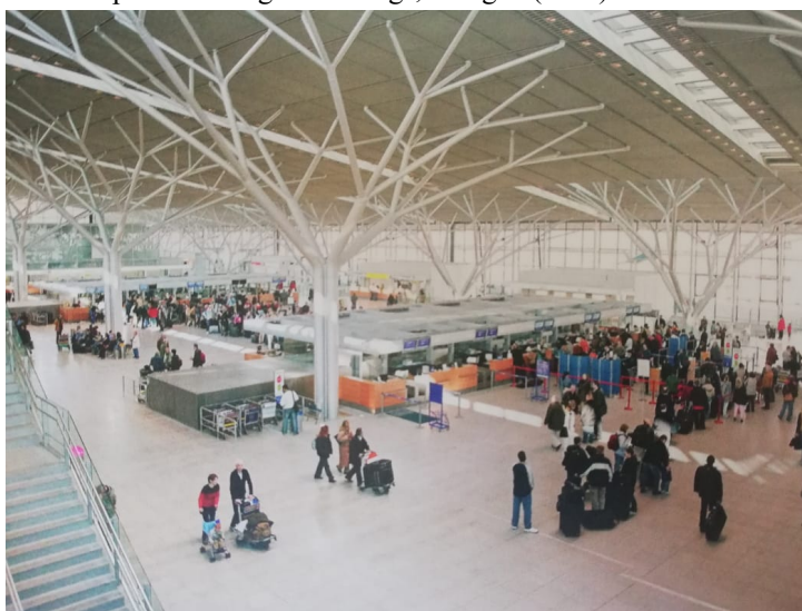
Fig. 5. Branched columns support the roof of Terminal 3 at Stuttgart Airport
