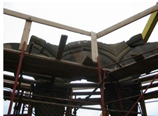
Fig. 14. Restoration of the southern altar arcade, 2002
